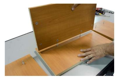
Install right hand and left hand sides by lining up the bolts to the cams. Turn cams using #3 screwdriver to fasten sides to shelf.
